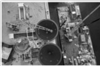
“Riga Bulk Terminal”.
